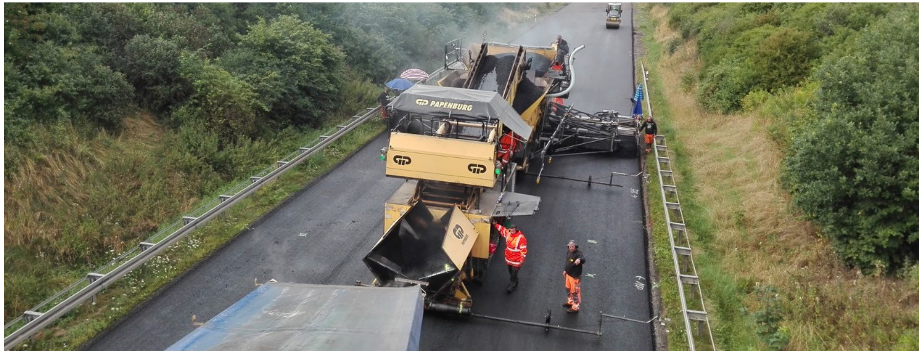
Within 10 days, 17,000 tonnes of compact asphalt was paved on the main road B180 near Rothenschirmbach.
