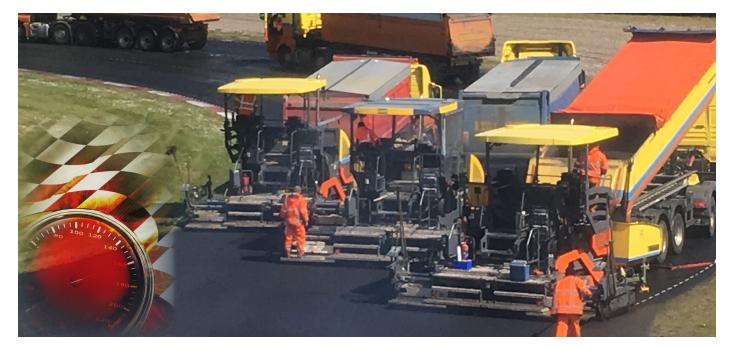
Just like on the highway, asphalt is a work of high precision. The current four centimeter asphalt surface must be removed first. A new layer is brought to a temperature of 160 degrees Celsius. In total, 14,500 tons of asphalt was required to pave the track. Unlike common roads, the curves require extra ordinary attention. "We have measured everything in detail. Every turn is different," says Bertram van den Brink, technical manager of De Jong Zuurmond who is responsible for work.
