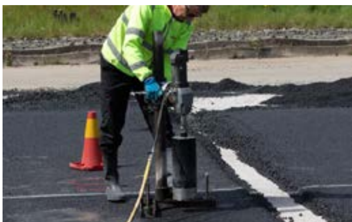
Figure 8. Coring in progress. 360 core samples were extracted during the in-house trials of the SEISMIC ASPHALT feature.
