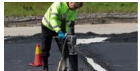
Compacting at the conventional fixed frequency.
