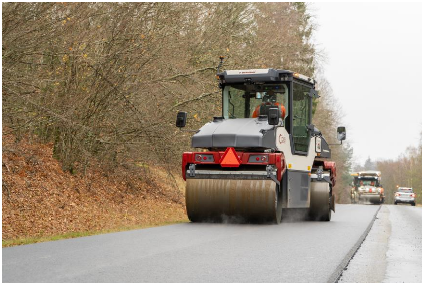
Caption: CX9C with SEISMIC ASPHALT jobsite
