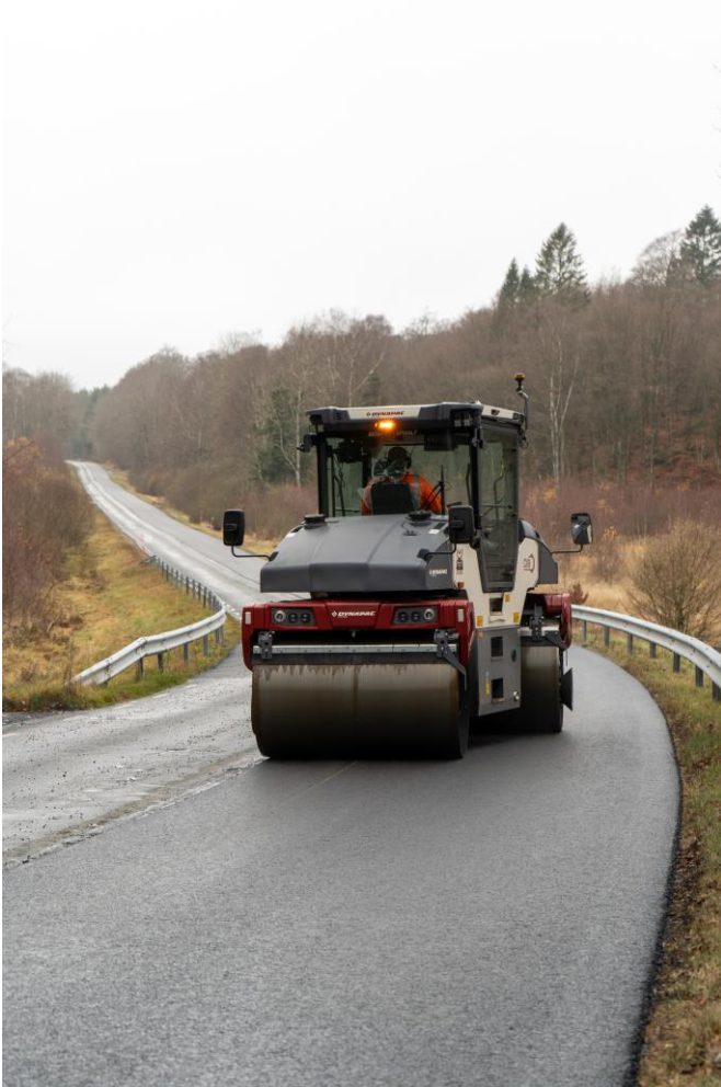
Caption: CX9C with SEISMIC ASPHALT jobsite
