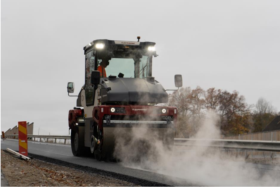
Caption: CX9C with SEISMIC ASPHALT jobsite
