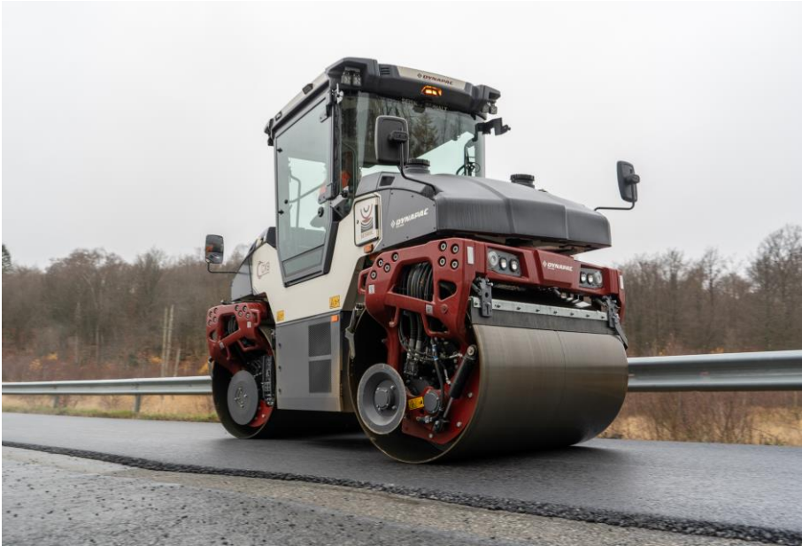
Caption: CX9C with SEISMIC ASPHALT jobsite
