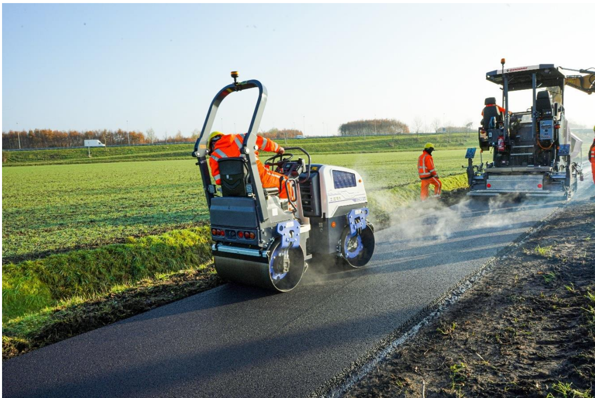
Dynapac electric SD1800We Citypaver and CC1000e Roller at work.
